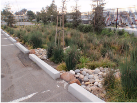
Include Stormwater Management BMPs
