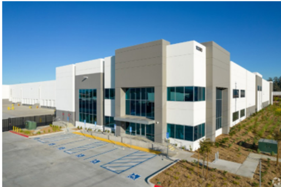
Typical Building Design with Concrete Wall Panels
